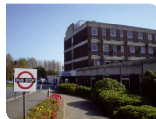
North Devon District Hospital
